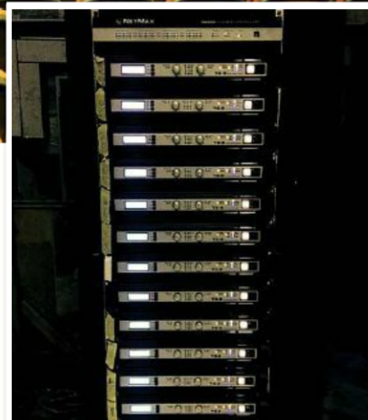
The NetMax N8000 controller installed in the rack alongside 17 TG-5 amps
